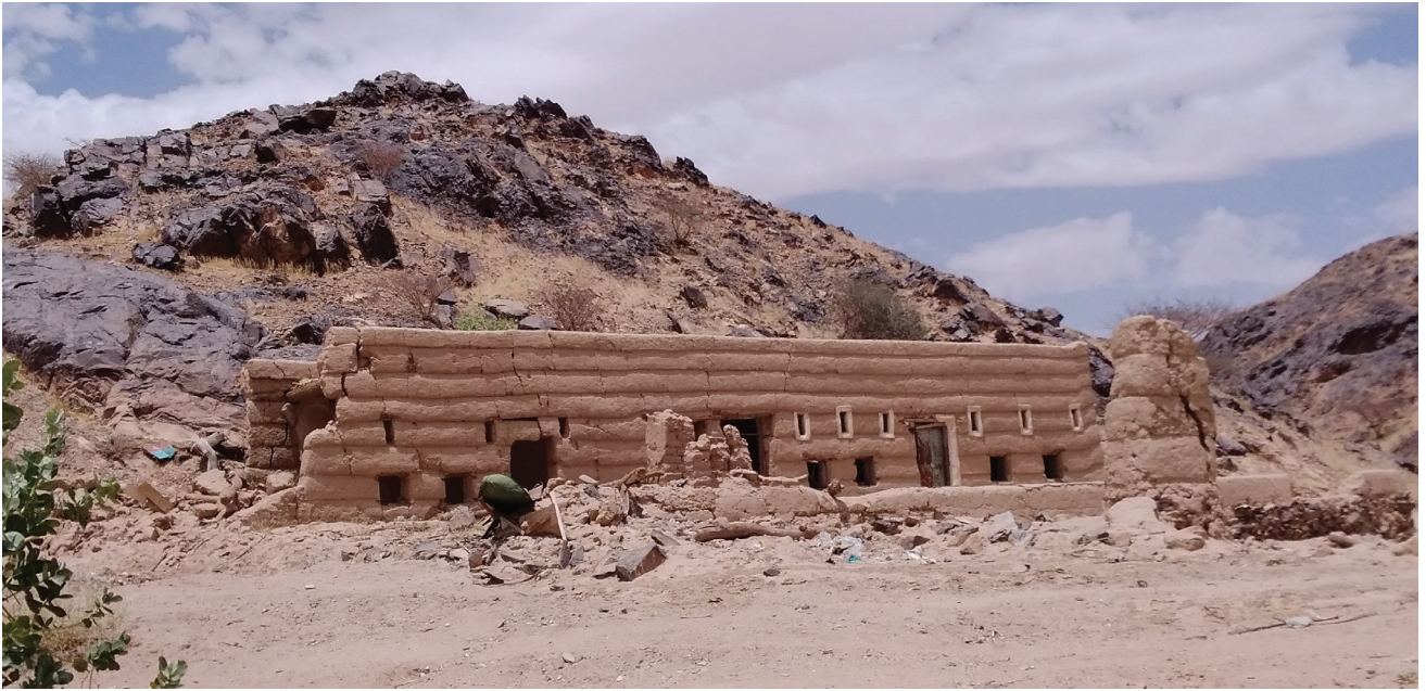
Ali Hamad's home in Barat Al Anan district, Al Jawf Governorate, before the Cash for House Rehabilitation Program.
