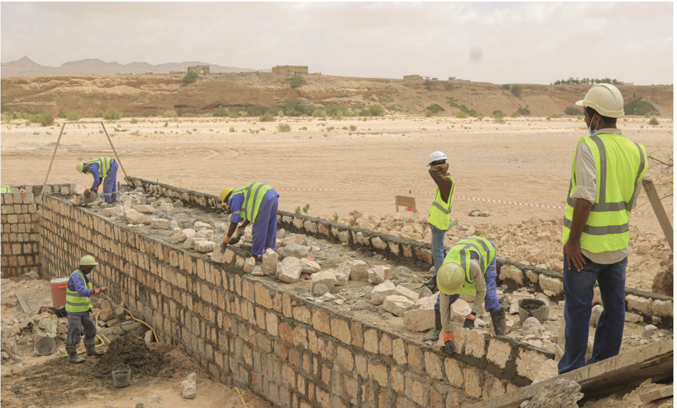
Muhammad, like many other workers who participated in this project, completed training on how to mix concrete, how to properly lay rocks and how to plaster walls before starting work onsite.
