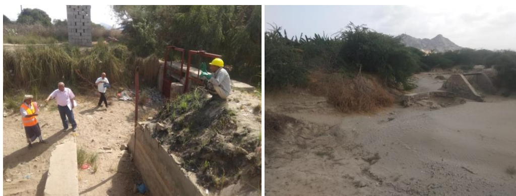
Photos 3.2a and 3.2b. Sediments and damages in irrigation canals and sub-canals, Khanfar district, Abyan | Photo Credit: UNDP, March 2022
