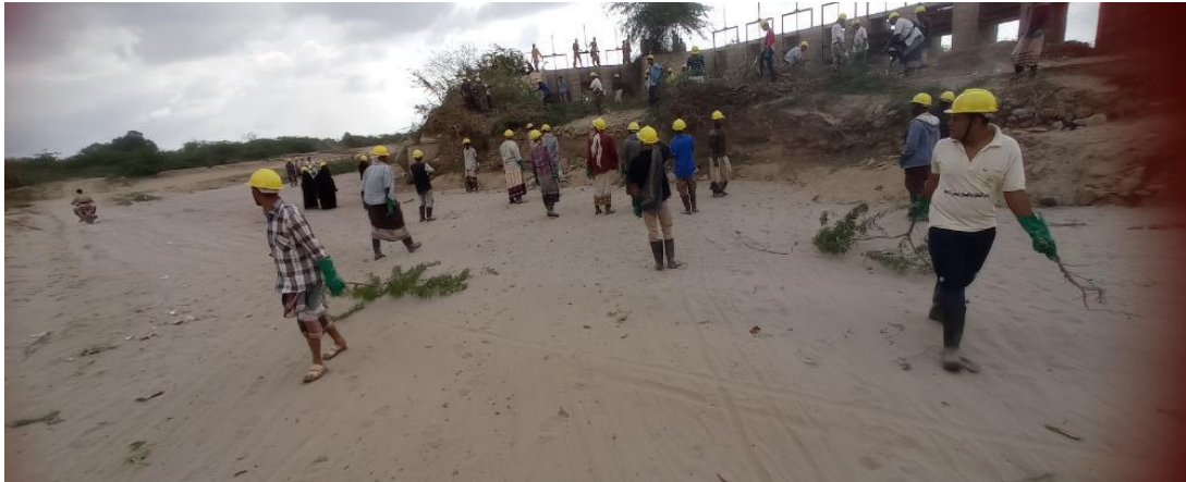
Photo 2.1 CfW for rehabilitation of irrigation infrastructures, Abyan | Photo Credit: UNDP, March 2022
